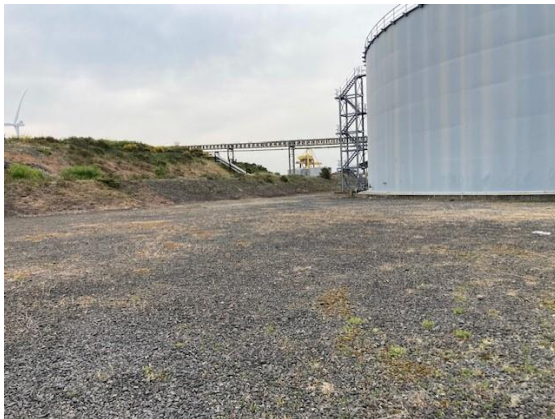
Photo 10.2: Building and surrounding gravelled surface within the Moneypoint Generating Station
