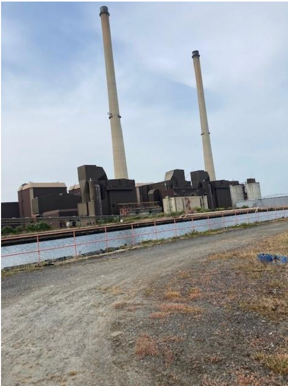
Photo 10.9: One of the water storage reservoirs in located within the Moneypoint Generating Station
